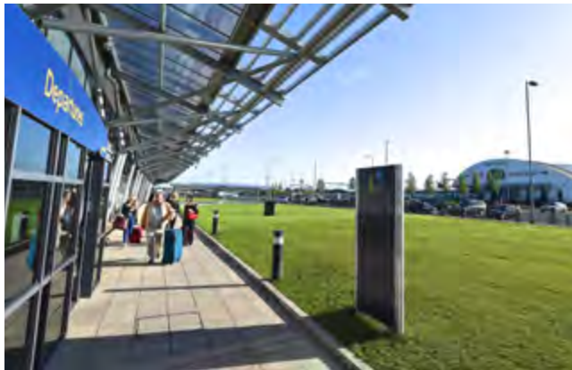
A short walk separates passengers arriving from the train station and the airport terminal.
